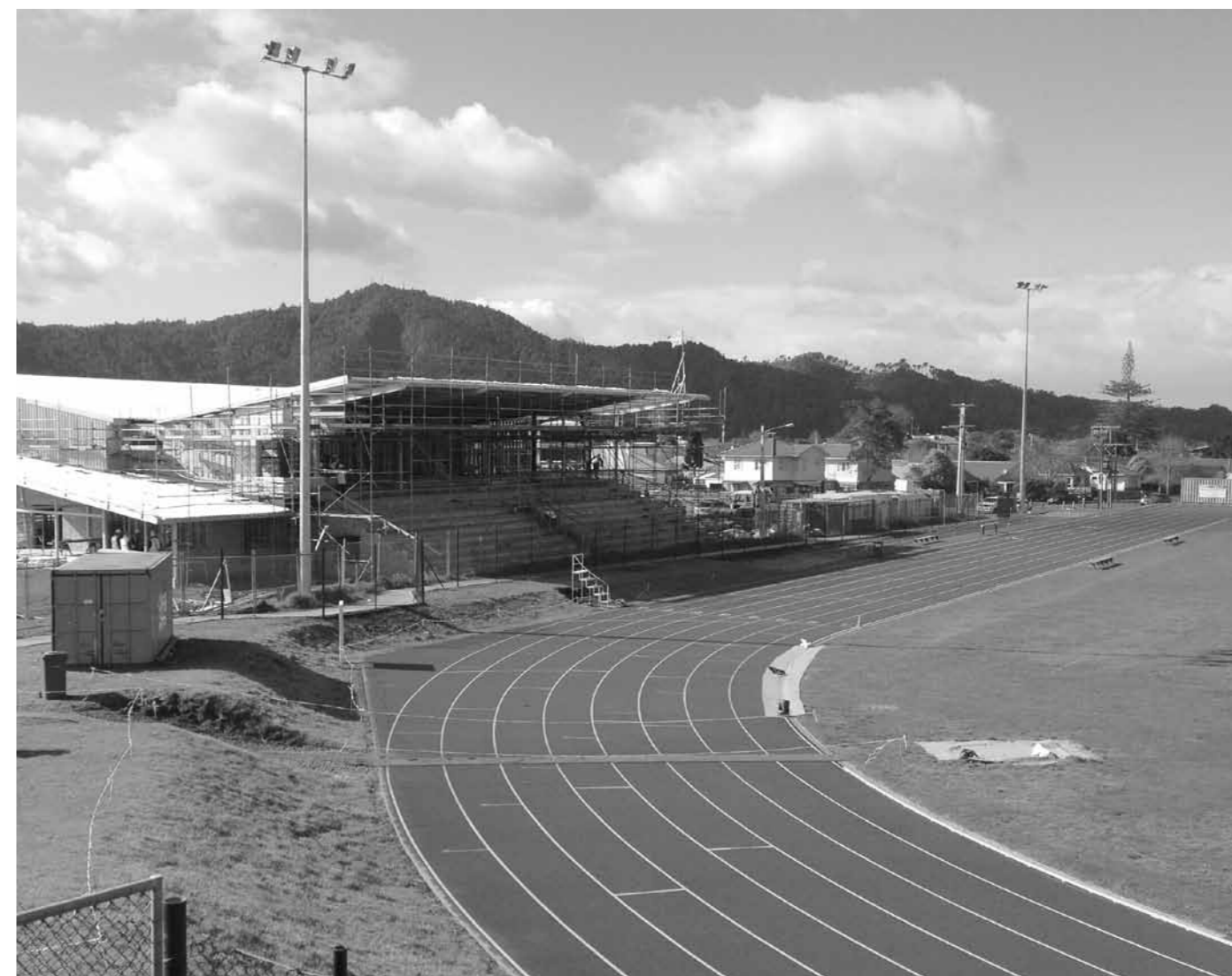
The new Northland Stadium Nears completion
