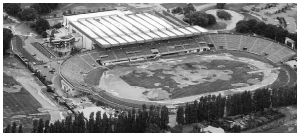
Aerial photo of damage
