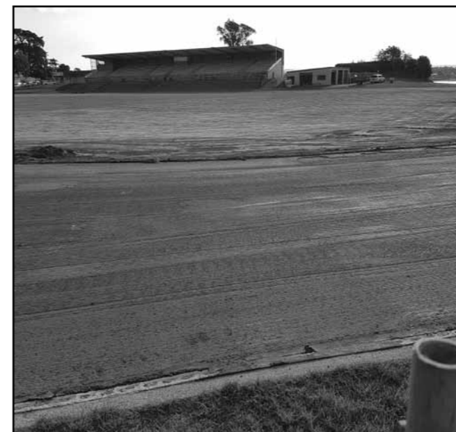
Work in progress on installing the new track at Tauranga Domain
