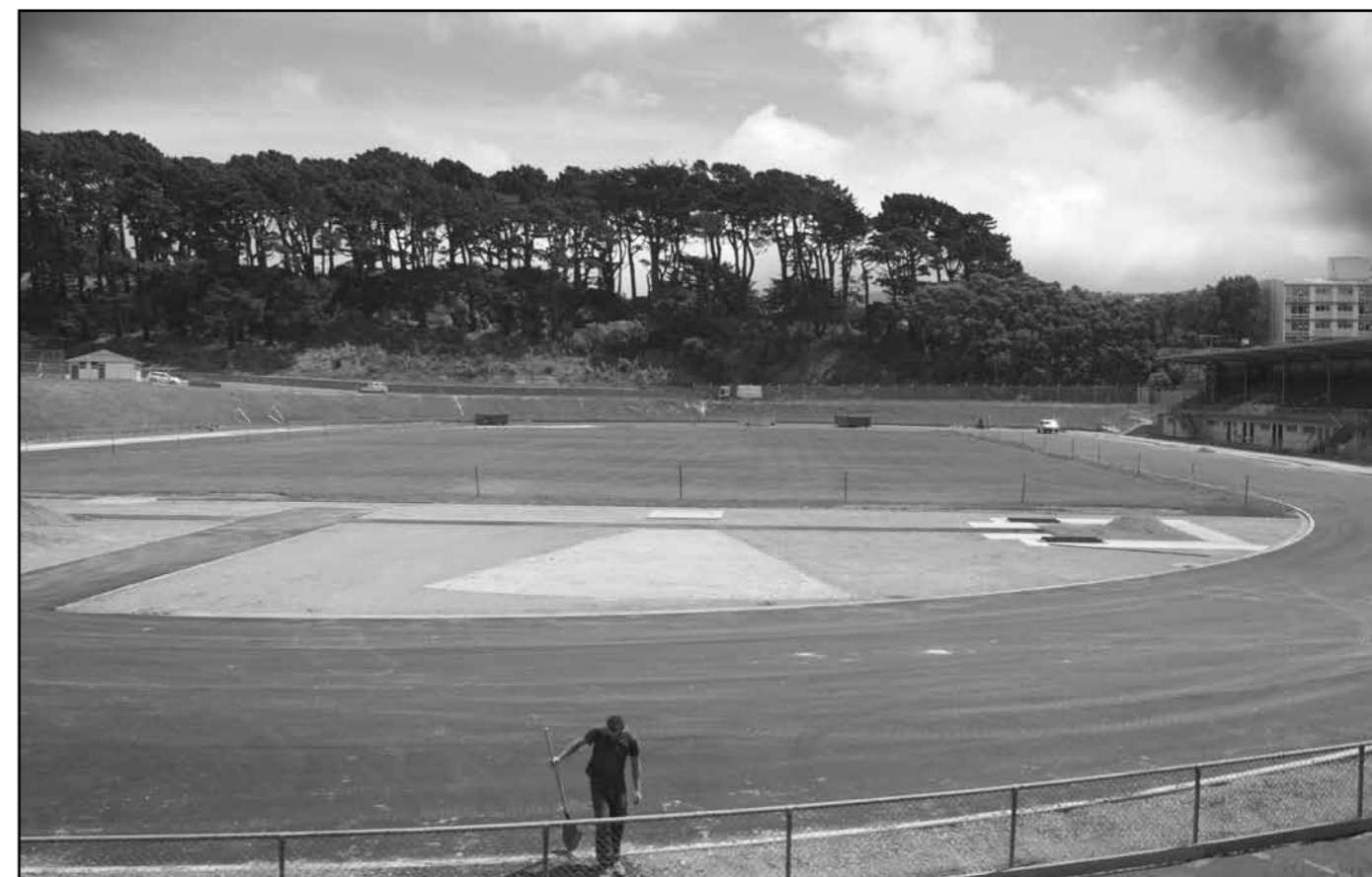
Newtown Park upgrade in progress
